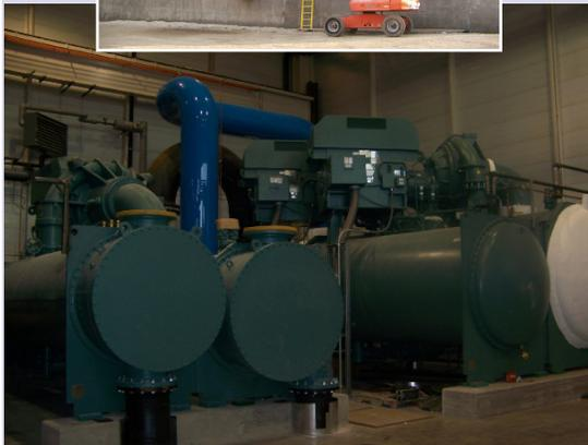
The new electric chillers installed as part of the Oak Street Chiller Plant ESCO project
