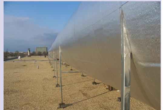
*The Basic Sciences Building features new fume hood exhaust ductwork and heat recovery systems*
